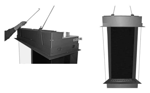
Fix the mantle iron to the rear wall with the bar set. Place the draw bars at an angle of about 60° (between the appliance and the wall). Level the mantle iron with the tension sleeves.
