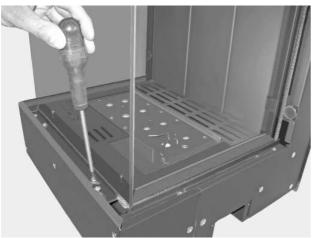
• Unscrew the strip at the front under the glass. Screws only need a couple of turns!
