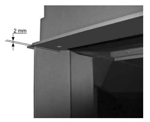
Keep a clearance of 2 mm between the mantle iron and the top of the side panels. The side panels should always be easily removable. Check that the mantle iron is at right angles to the side panels, both left and right. Put ceramic felt on the top of the mantle iron, before laying bricks or using other non-flammable structural materials.
