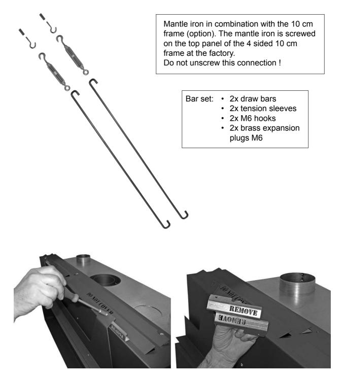
First remove the 2 mantle iron transport-spacers "REMOVE" **Note!** Temporarily support the mantle iron, so that it does not fall forwards.
